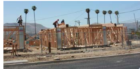
Construction at Central Station in Fillmore
